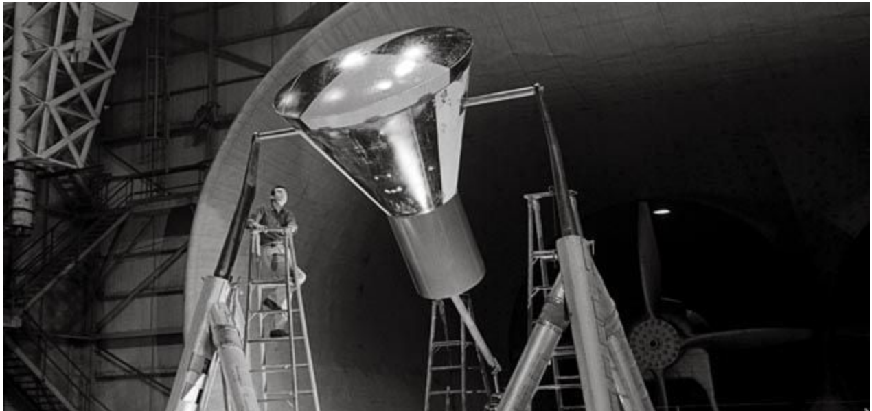
The Mercury space capsule during a 1959 wind tunnel test. NASA Langley Research Center
