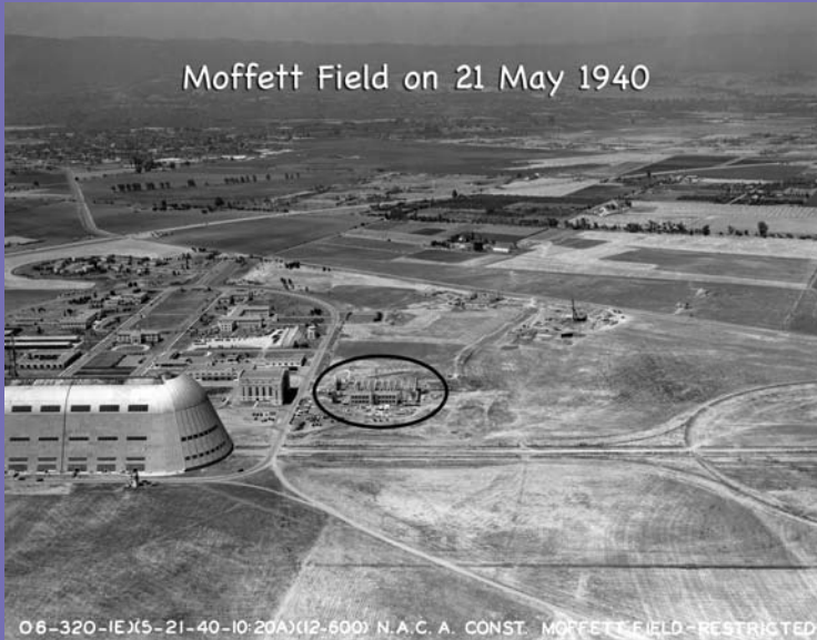
Moffett Field on May 21, 1940. Groundbreaking for the first permanent Ames building (now N210) was in late February.
