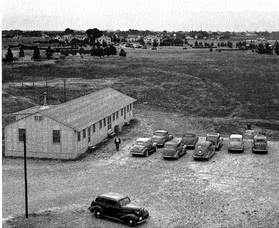
January 1940. The first building erected at Ames, the construction shack served as headquarters for the engineers and crews fighting California's winter mud as they laid out and built an aeronautical laboratory.
