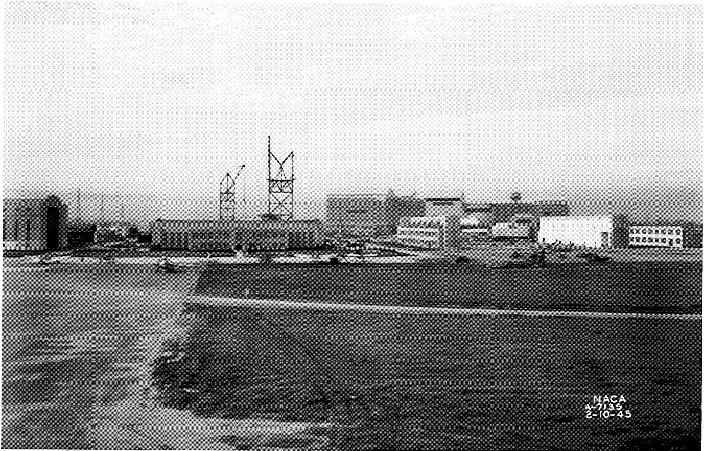
Figure 30 New flight research hangar under construction circa 1945.
